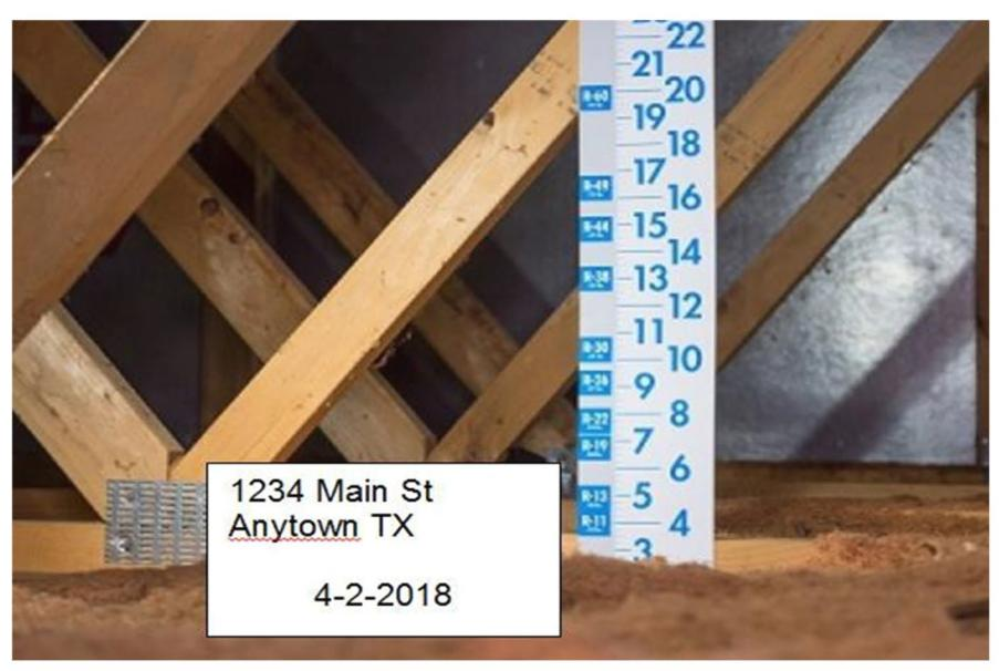
A photograph showing wooden roof trusses and insulation. A vertical blue ruler is placed against the insulation to measure its thickness. A white identification card is overlaid on the image, containing the text: 1234 Main St, Anytown TX and the date 4-2-2018. |
