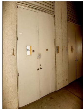
Pictured: Walk-in Vault
