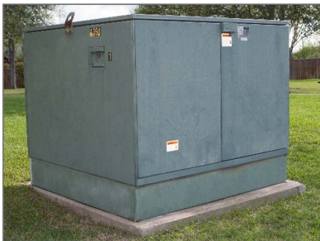
Pictured: Pad Mounted Switchgear (left); Switches (right)
