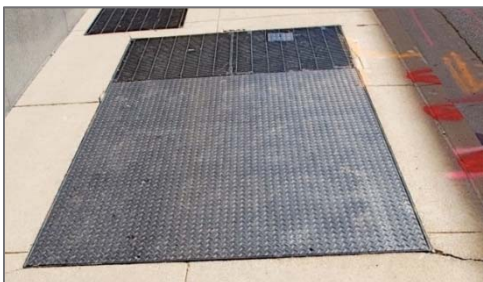
Pictured: Sidewalk Vault
