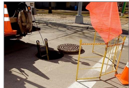
Pictured: Underground Manhole
